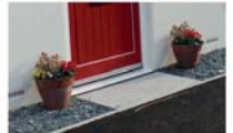
Where the building line forms the edge of the public realm, careful consideration is needed as to how the curbside of the property is defined.
