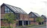
Typically detached barn like structures. Use of stone and weatherboarding with an emphasis on vertical rhythm.
