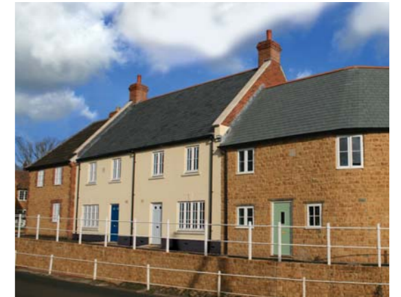
A harmony of tiles, stone, slates and render
